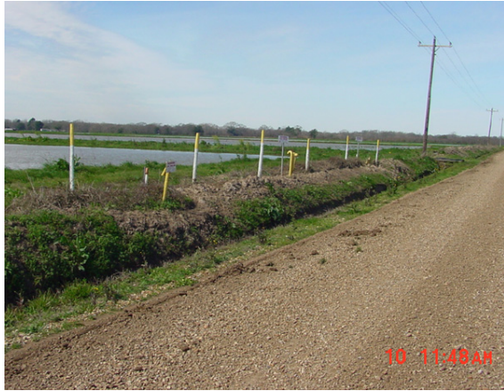
Figure 2.2.2 Well labeled warning posts
