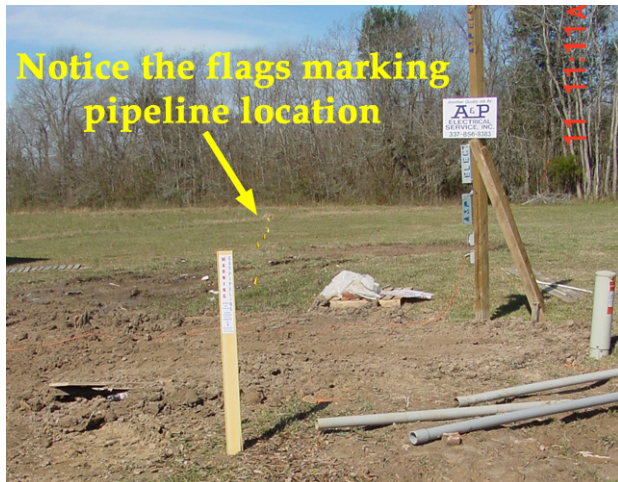
Figure 3.2.6b Efforts to mark pipelines
